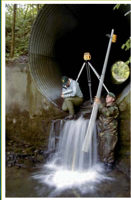
Culvert assessment/C. Alexander
